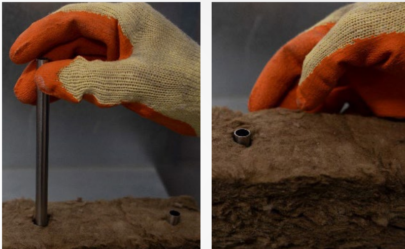
Figure 08 – Installation of anti-compression sleeves
