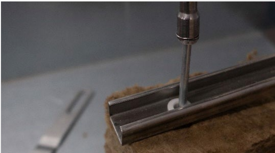
Figure 10 – Installation of fasteners for retention of wall-tie system to mild structural steels
