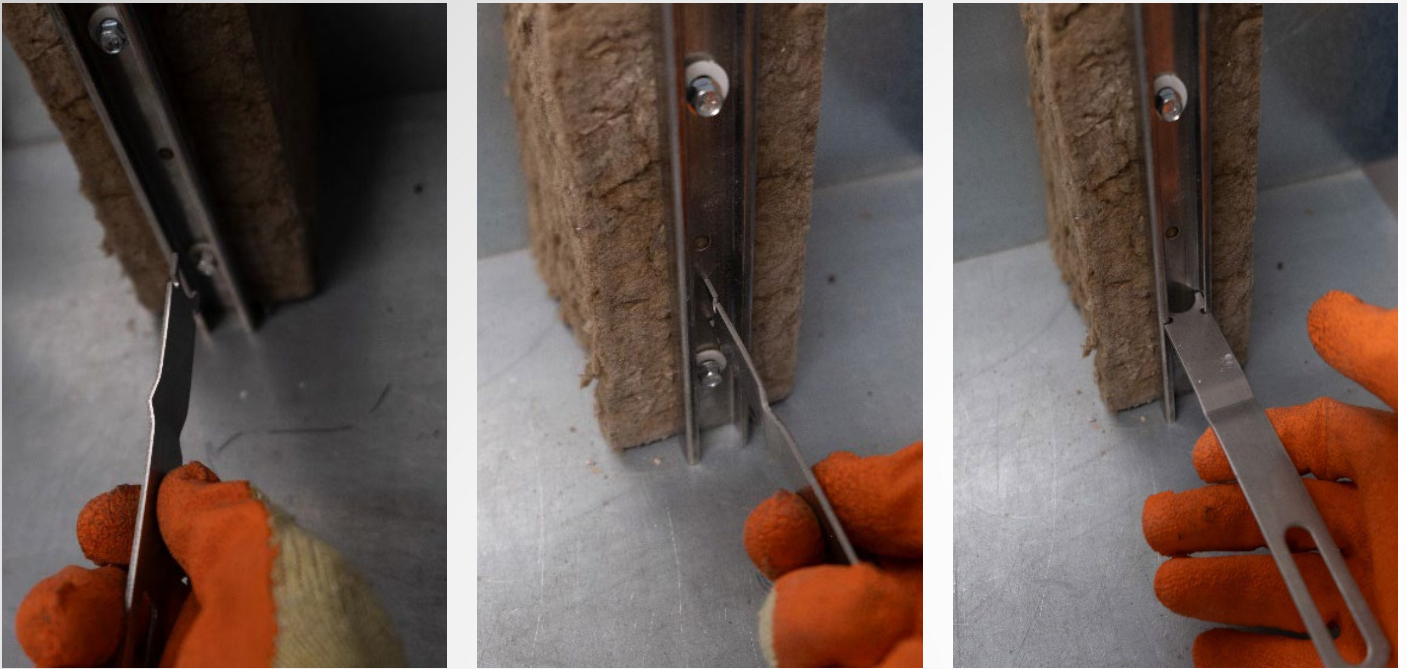
Figure 13 – Installation of wall-ties into retention channel
